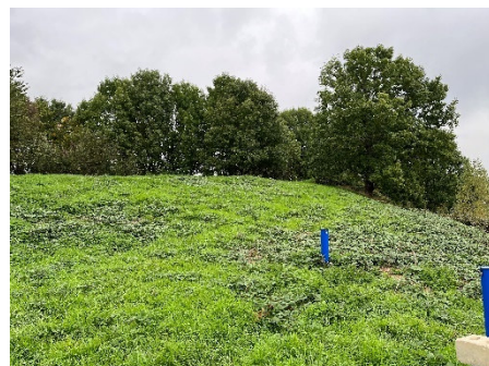
Bodendepot am Grubenrand
